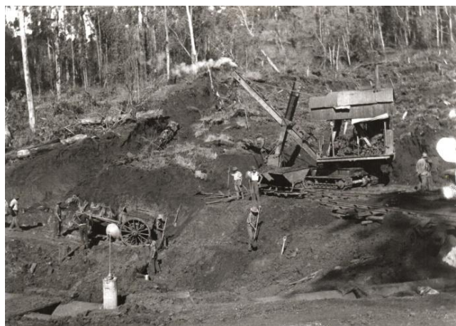
Workmen with steam shovel and cart repairing the Silvan Aqueduct after the landslide, January 1935. Photo Cedric (Louise) Hordern.
