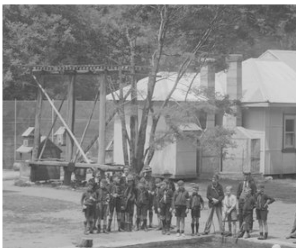
Close-up of the timber frame at the Recreation Camp. The consensus is 'tank stand'.
