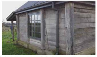
'Elm Cottage' showing the horizontal slab construction.
