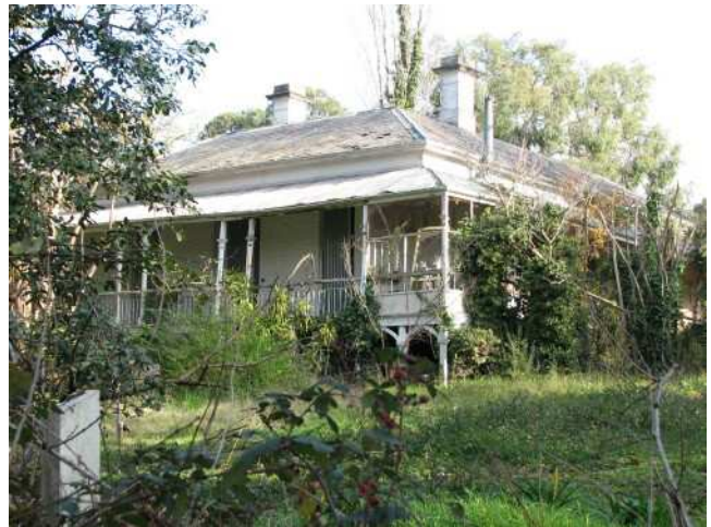
The Manor House from the north-east. Photo Kevin Phillips.
