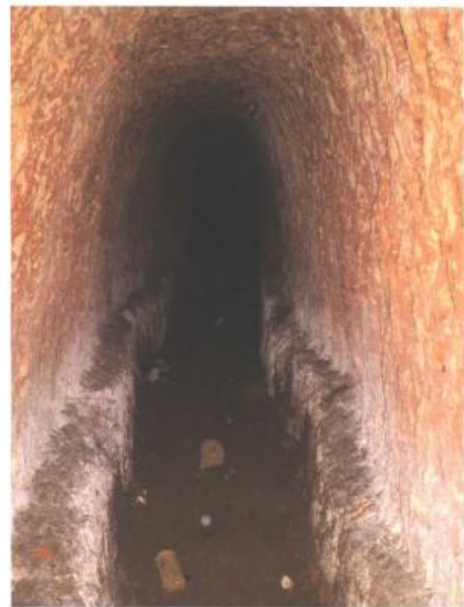
Tunnel at Kalorama, purpose unknown
