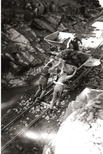
Workers on the Aqueduct. From The Hordern Collection. Photo: Cedric Hordern.
