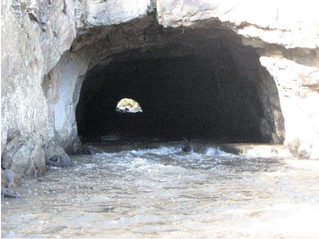
Light at the end of the Pound Bend Tunnel.
