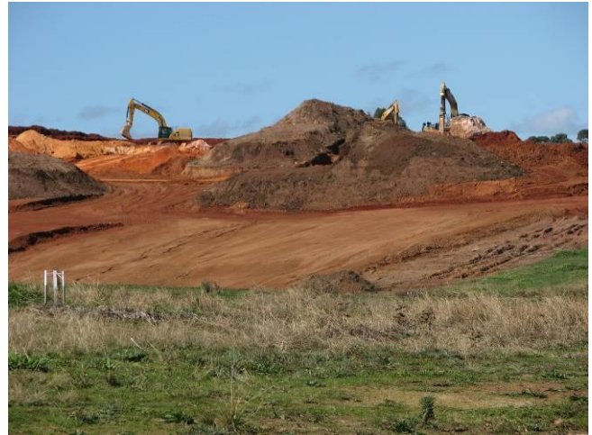
Above, earth-moving machines at Red Hill, on the former Cave Hill Estate. Photos Kevin Phillips.
