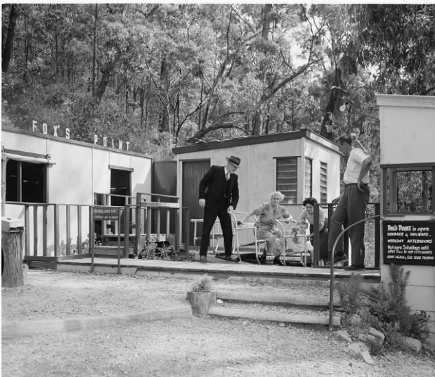
Above, the control level. Neil Foxcroft is the tall man standing at right, next to the control room. Victorian Railways Collection, State Library Victoria.
