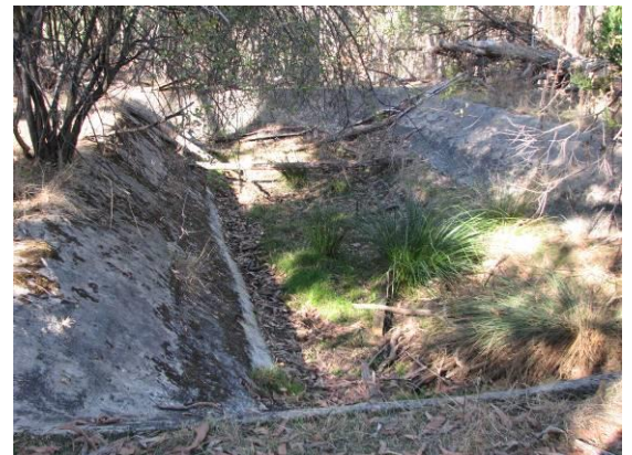
Water storage tank
