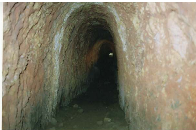
Inside the tunnel, looking back towards the entrance.
