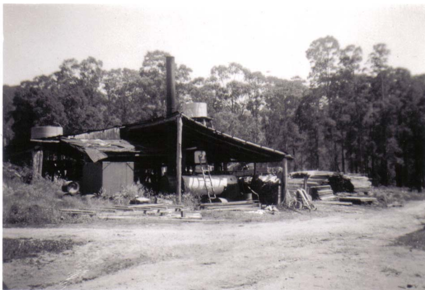
Above, the sawmill boiler house with water tank, chimney, boiler and stacks of sawn timber. Photos courtesy Beryl Taylor.
