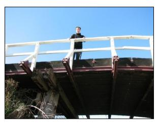
Greg on the bridge. The wooden pylons, bent rail track decking and cross-pieces can be seen. Photos Kevin Phillips.
